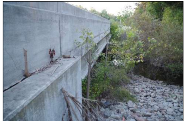
Photo 36. PC Pkwy Bridge over McChune Branch
