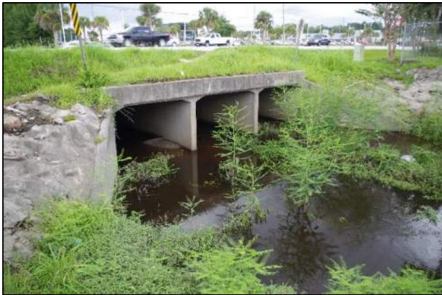
Photo 9. Ashley Phosphate Road Upstream
