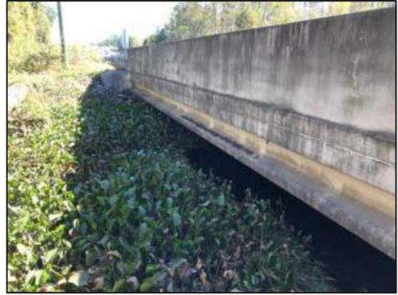
Photo 62. Hwy 78 Bridge Downstream
