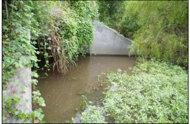
Photo 32. Culvert PC Pkwy Downstream
