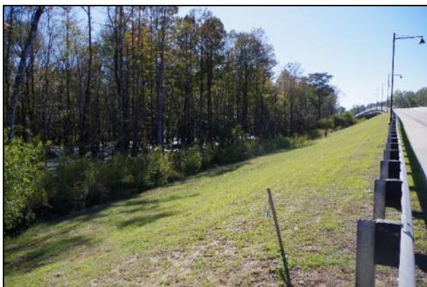
Photo 53. Wetlands Upstream Weber Blvd
