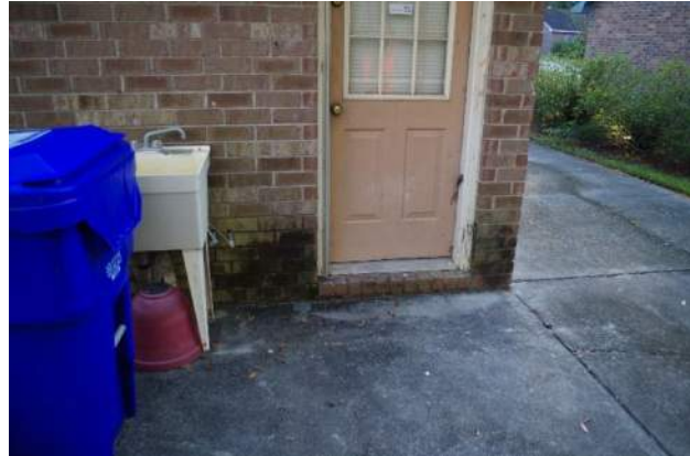
Photo 7. Finished Floor above Ground Surface
