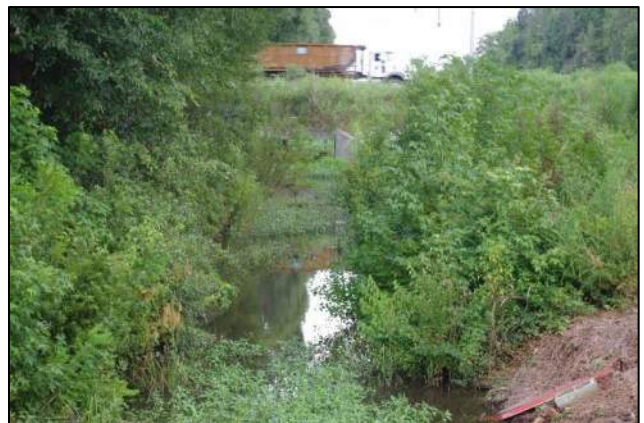
Photo 30. Ditch and Box Culvert Facing PC Pkwy
