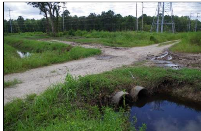
Photo 22. Upstream Utility Road Crossing 8/25/17
