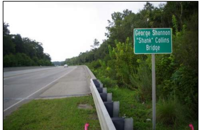
Photo 34. Palmetto Commerce Pkwy Long Bridge
