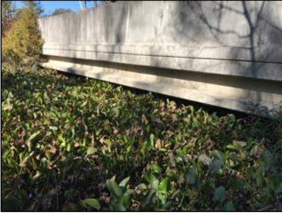
Photo 61. Hwy 78 Bridge Upstream
