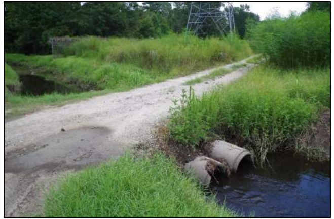
Photo 20. Downstream Utility Road Crossing 8/25/17
