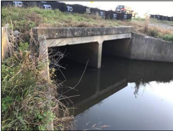
Photo 1. Dorchester Road Downstream
