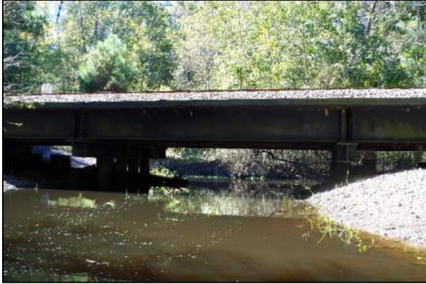
Photo 49. McChune Branch Downstream Railroad Bridge
