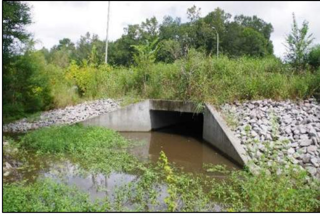
Photo 31. Culvert PC Pkwy Upstream
