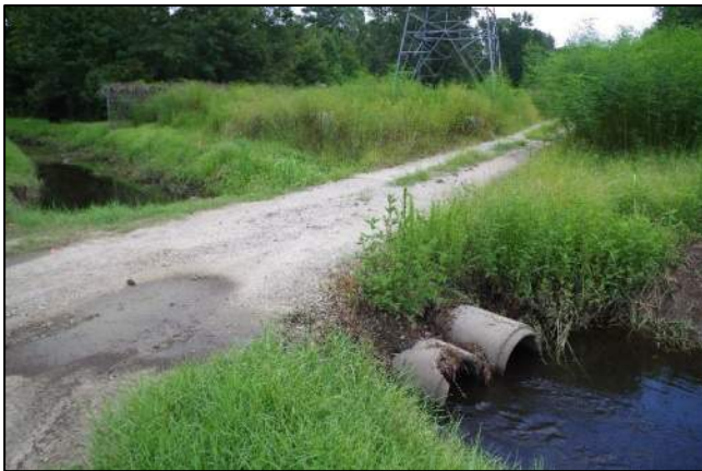
Photo 21. Downstream Utility Road Crossing 8/25/17
