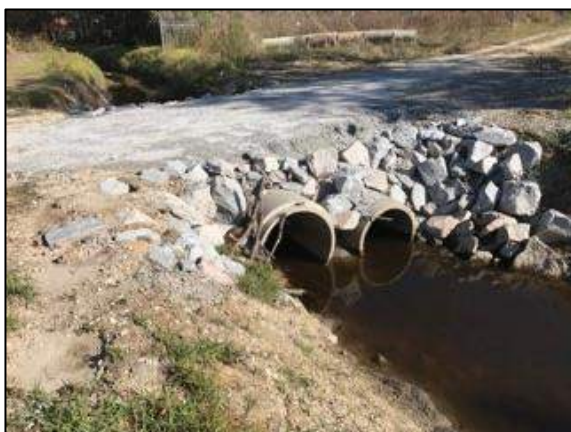
Photo 23. Utility Road Crossing Downstream 11/2017
