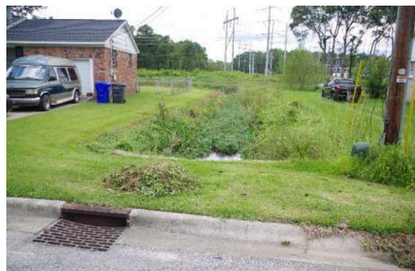
Photo 2-2. Drain Inlet and Ditch on Peppercorn Lane
