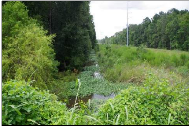
Photo 33. Ditch Downstream PC Pkwy Box Culvert
