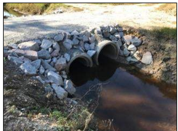
Photo 24. Upstream Utility Road Crossing 11/2017
