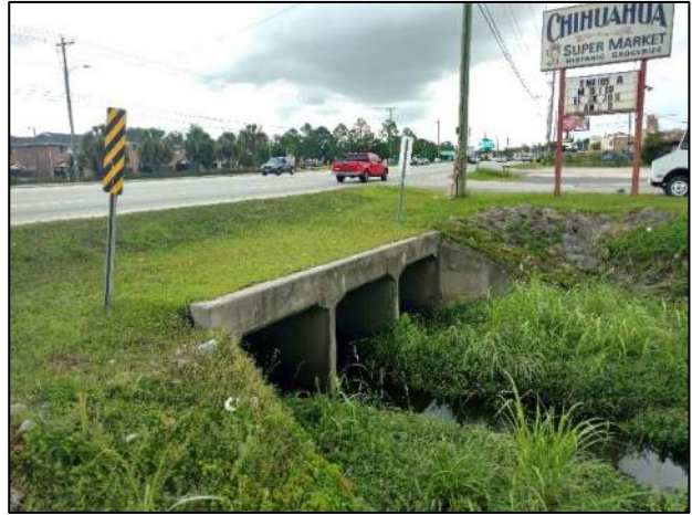
Photo 8. Ashley Phosphate Road Downstream
