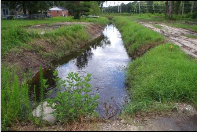
Photo 19. Downstream Utility Road Crossing 8/25/17
