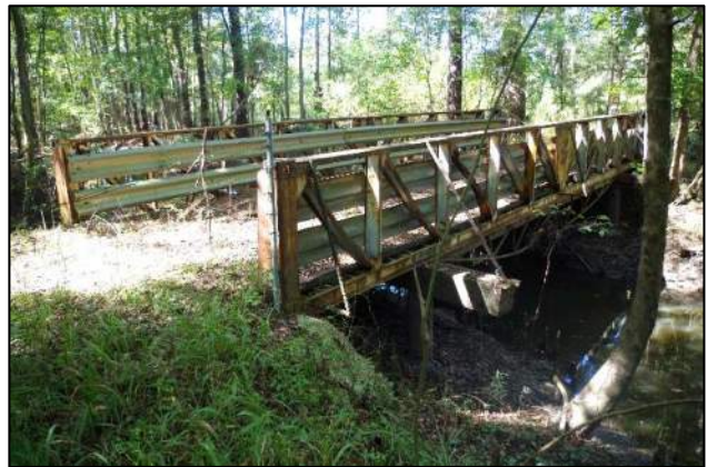
Photo 40. McChune Branch Wood/Metal Bridge
